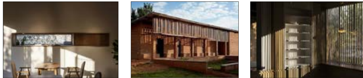
Some examples how similar effect can be achieved in a built form.
