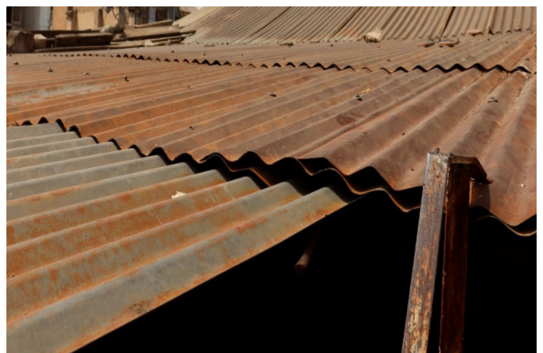
Above: Roof of House
