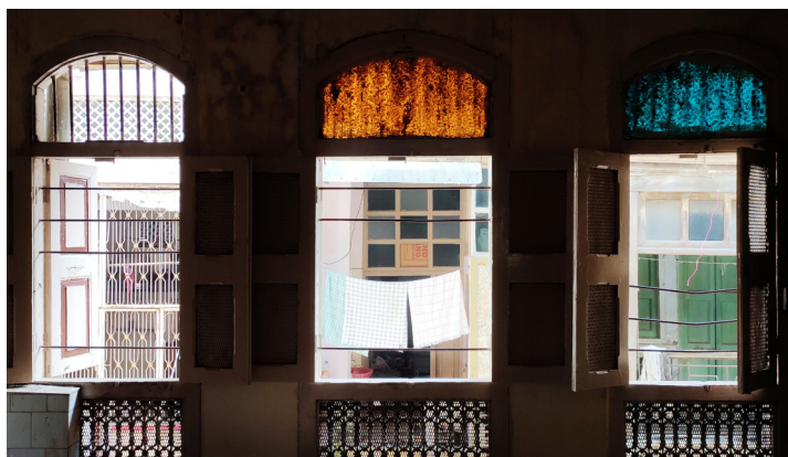
View from the first floor
