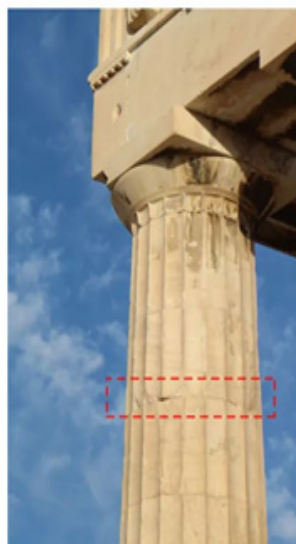
DORIC COLUMN AT THE PARTHENON, ATHENS (RED RECTANGLE IS WHERE THE STONES ARE RESTED ONTO ONE ANOTHER)
