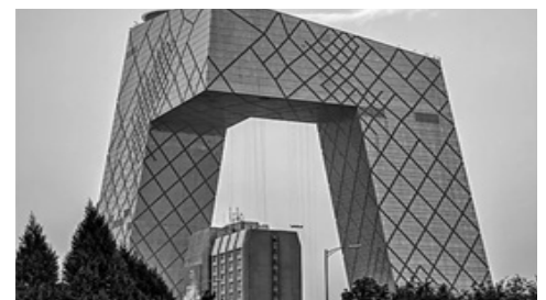
VIEW OF CCTV HEADQUARTERS WITH THE FALSE STRUCTURAL DIAGRID ON THE FACADE, OMA (2012)
