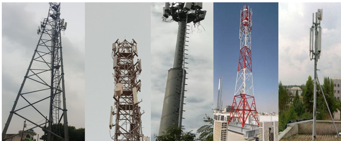
(a) Ground-Based Tower (GBT), 3-Legged (b) Ground-Based Tower (GBT), 4-Legged (c) Ground-Based Mast (GBM) (d) Roof Top Tower (RTT) (e) Roof Top Pole (RTP)
