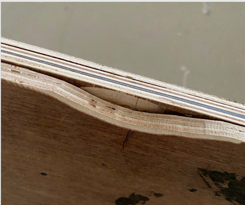
A depression to make it easy to pull the slider out with hands.
