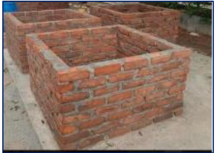
(b) Bricks wall of pond
